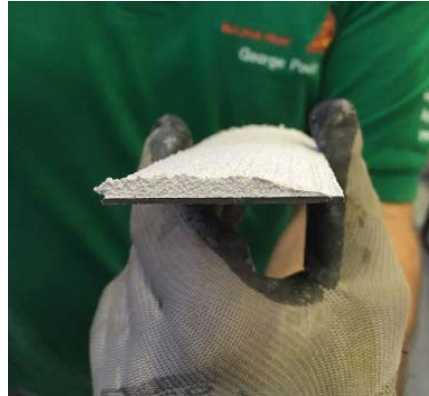
Figure 4.1: Sikadur 30 applied onto Sika CarboDur plate
