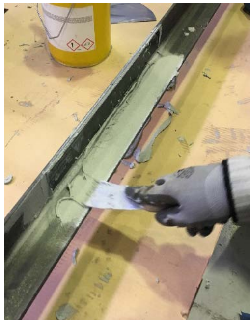
Figure 4.2: Application of the resin on the prepared steel member
